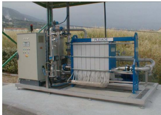
Fig. 12.10 Plate and frame module in waste water system
